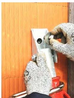
FIGURE 2: BRIQUE A DOUILLE M16
